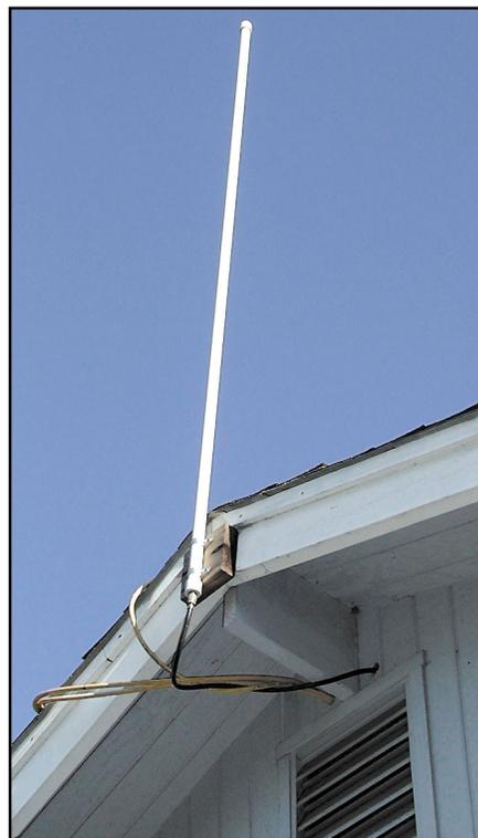
**Figure 5—The completed antenna mounted to the roof.**
